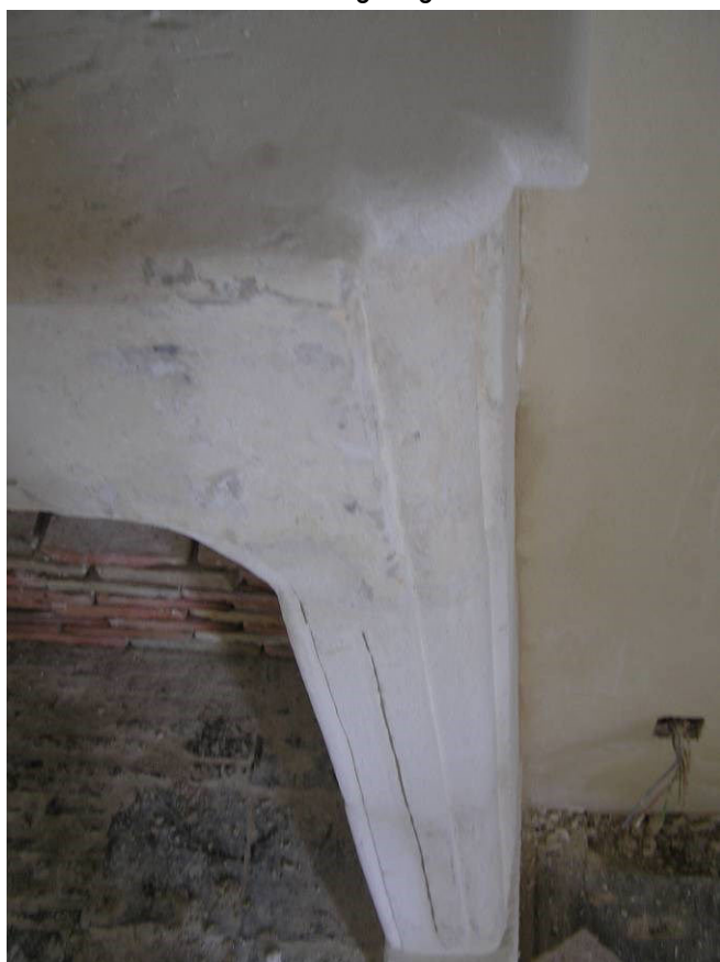
While renovating stage
