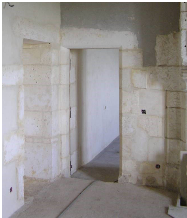
While renovating stage
